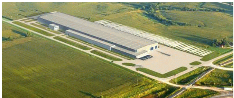
TPI Composites Wind Turbine Facility at Newton, Iowa
